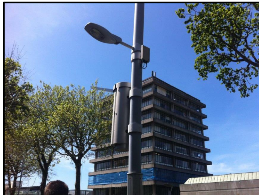
Small Cell Equipment and separate Antenna within Auckland CBD
