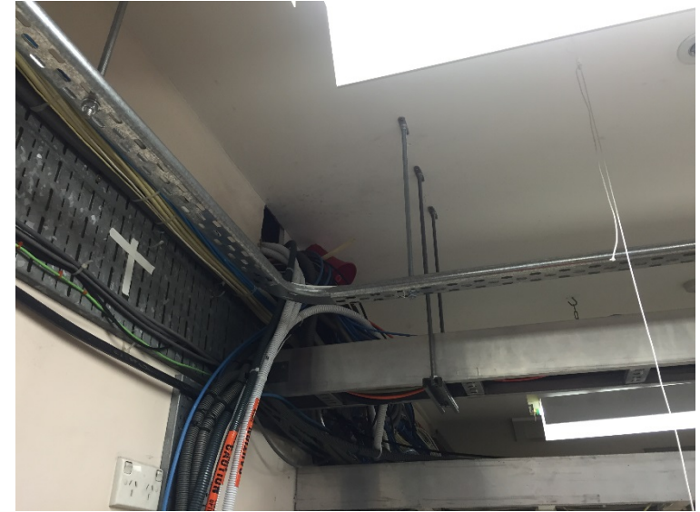
Existing access hole and cabling
