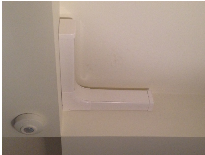
On wall corner capping
